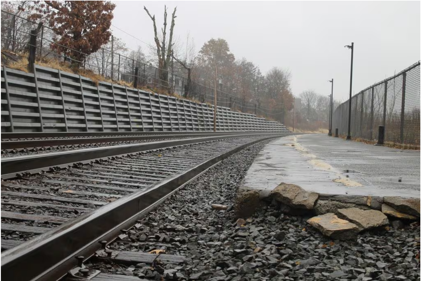
Rebuilding the crumbling commuter rail stations in Newton would cost more than $170 million. HEATHER HOPP-BRUCE
