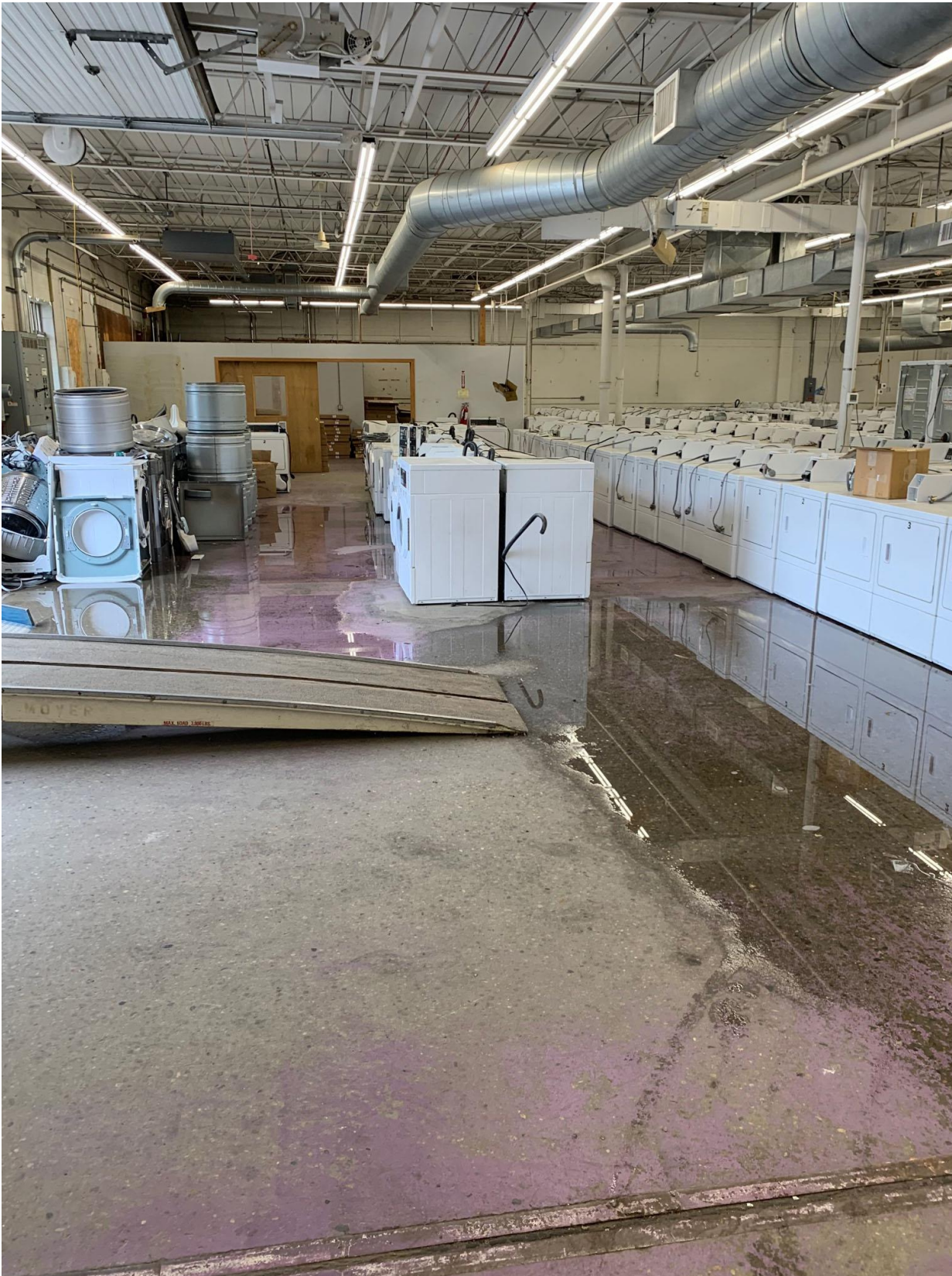
June 2020 (Automatic Laundry - flooding reached equipment area)
