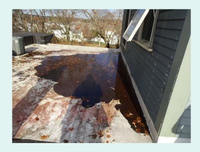
Existing roofs must be replaced. The new roof insulation will be increased to R-50, and the new roof will be a white TPO. The existing apartment air conditioning condensers must be removed and all 35 units replaced. These will be replaced with heating/cooling heat pumps to reduce green house gas emissions. Three gas fired Roof Top Units (RTU's) that cool the common areas will be replaced with higher efficiency equipment.
