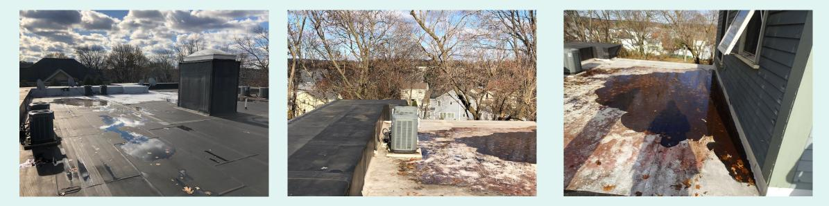
Existing roofs must be replaced. The new roof insulation will be increased to R-50, and the new roof will be a white TPO. The existing apartment air conditioning condensers must be removed and all 35 units replaced. These will be replaced with heating/cooling heat pumps to reduce green house gas emissions. Three gas fired Roof Top Units (RTU's) that cool the common areas will be replaced with higher efficiency equipment.
